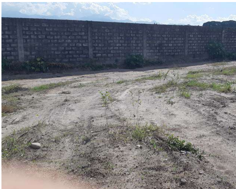
Fig. 4: Photo of site as of June 17, 2020
