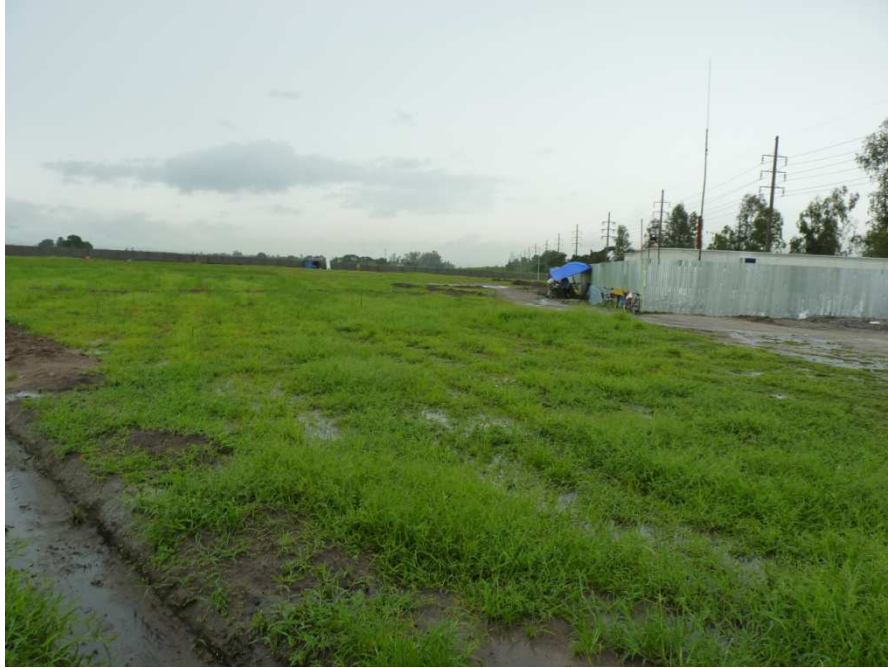
Fig. 5: Northern part of the site with transmission line and construction site facilities (right)
