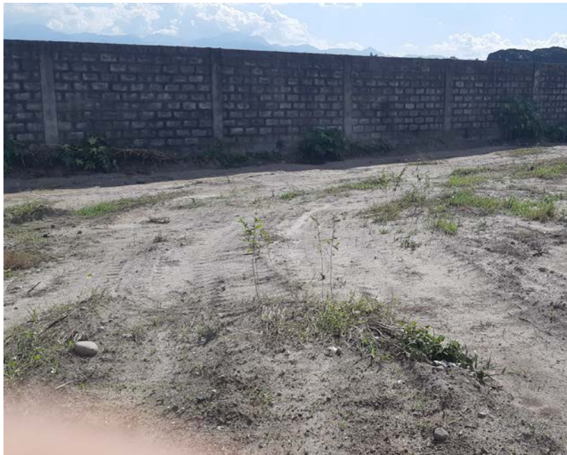
Fig. 4: Photo of site as of June 17, 2020
